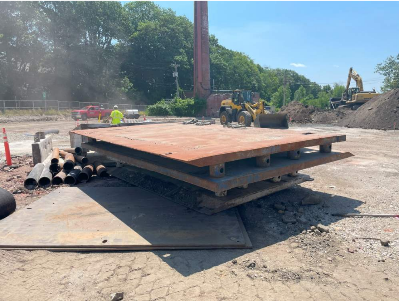
Photo 1. Trench Box removed from site observed.
