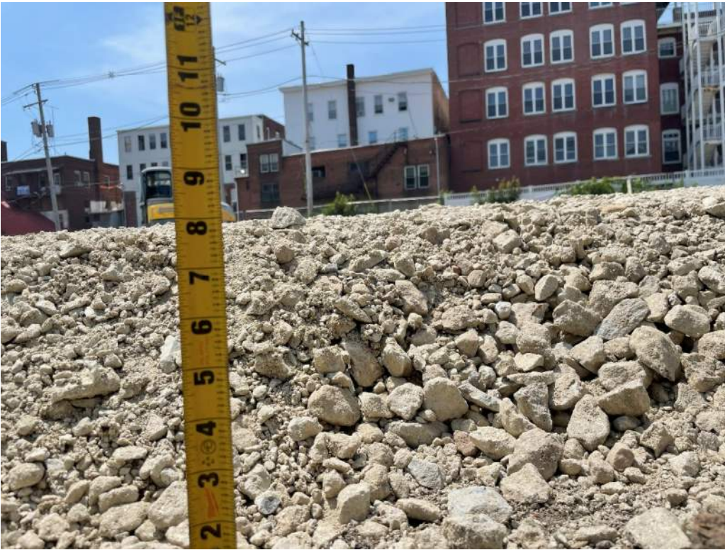
Photo 4. Compacted processed gravel subgrade at 8 inches.
