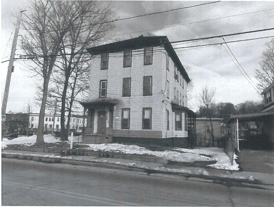
Front and South Side of the Building
