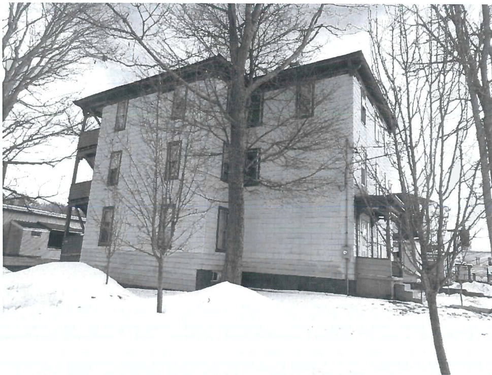
North Side of the Building
