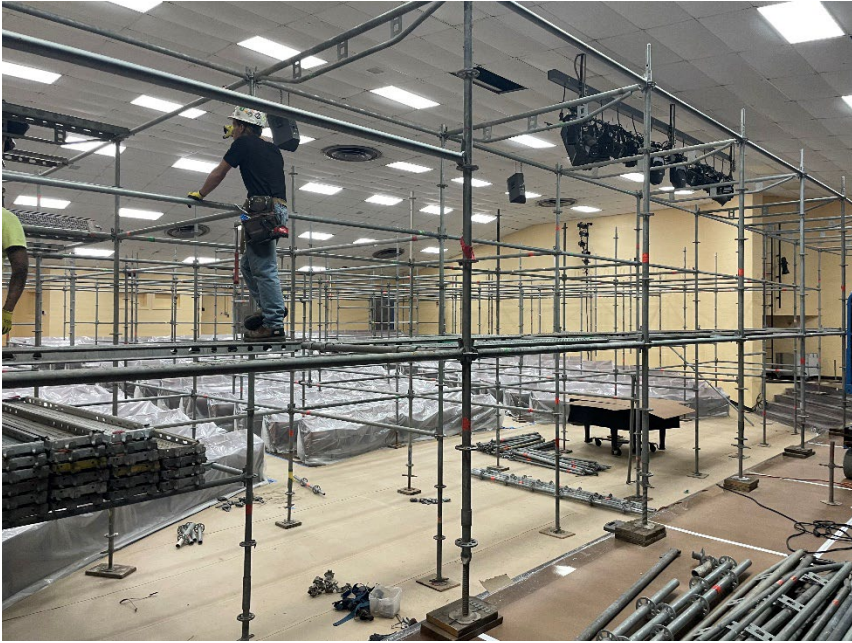
Scaffolding in GHS Auditorium being installed.
