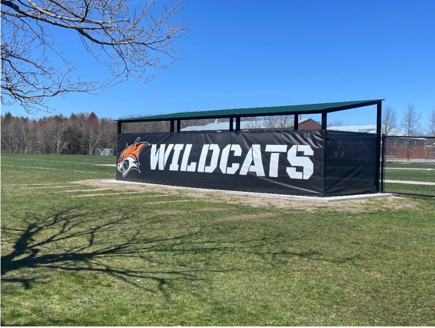
WILDCATS wind screens on the new dugouts
