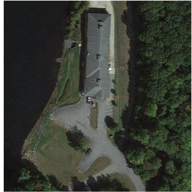
Crystal Lake Water Treatment Facility
