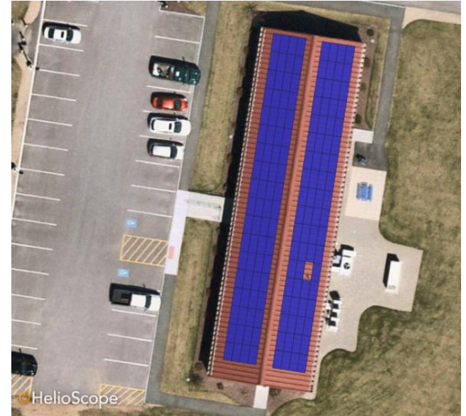
Gardner DPW (South) – 68.6kW
