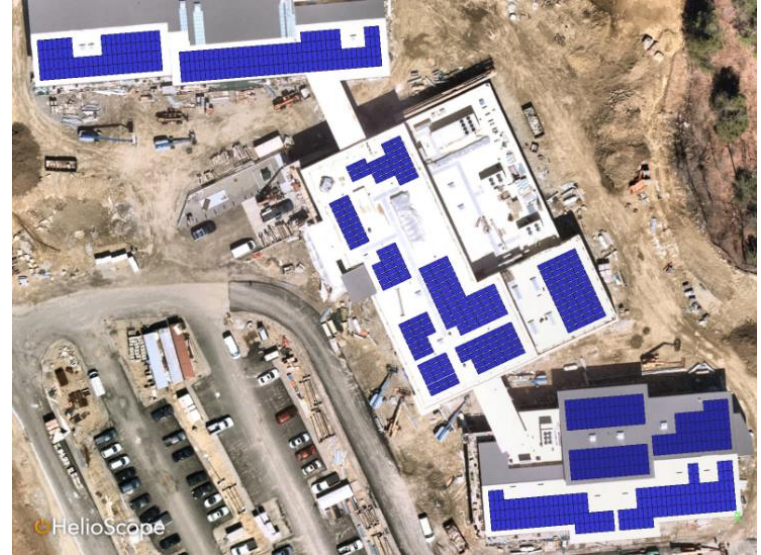
Gardner Elementary School – 372kW
