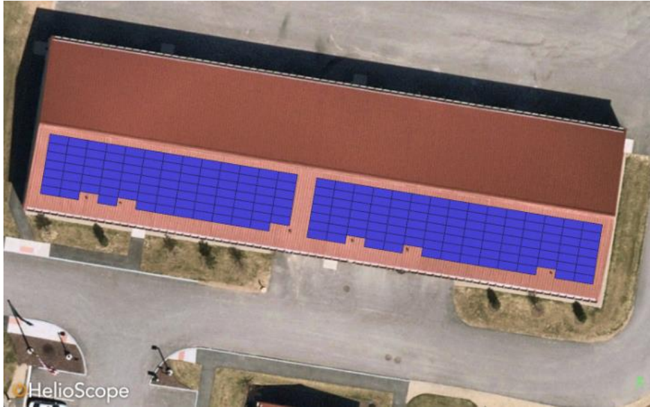
Gardner DPW (North) – 91.2kW
