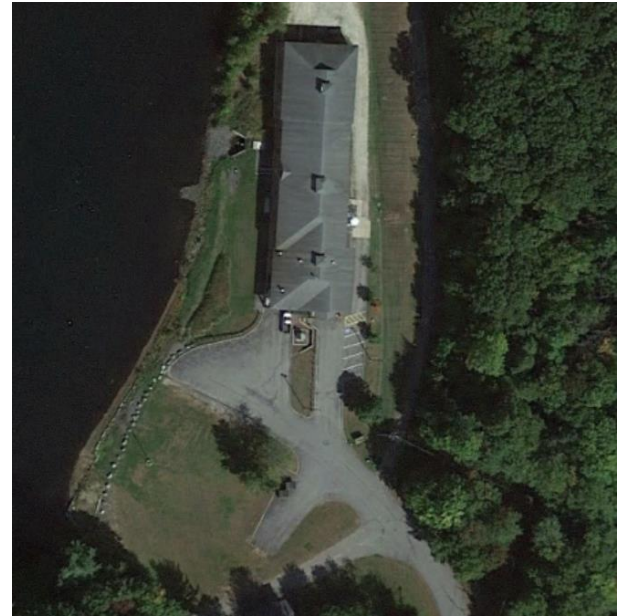
Crystal Lake Water Treatment Facility
