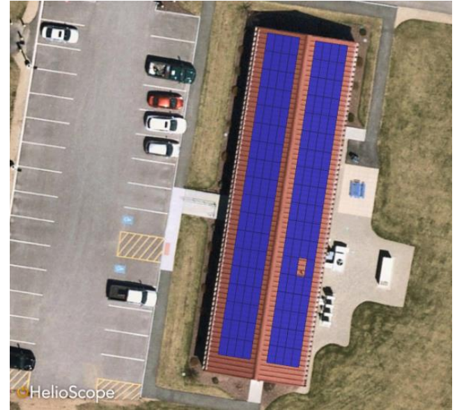
Gardner DPW (South) – 68.6kW
