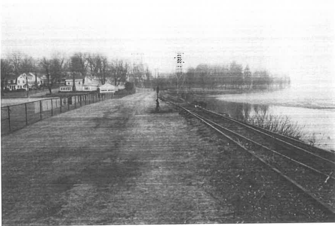
Photo B1: View of the dike crest looking towards the right abutment.
