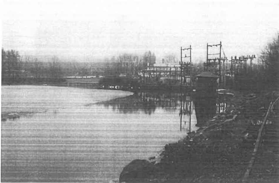
Photo B3: View of the dike upstream slope from right abutment.
