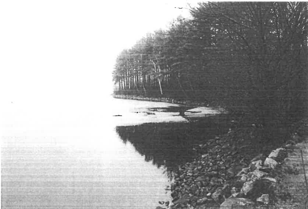
Photo B12: View of the left abutment
