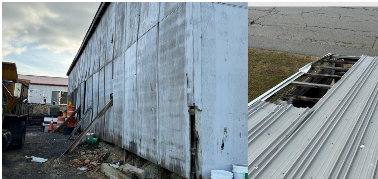
Figure 3: Existing Salt Shed, West facing wall with supports and Southeast Corner of Roof with hole
