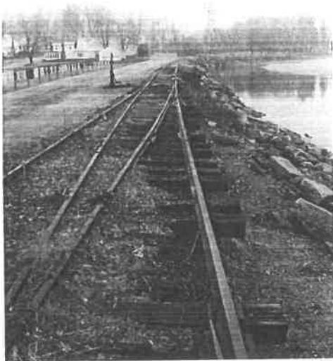
Photo B2: View of the dike crest looking towards the right abutment.
