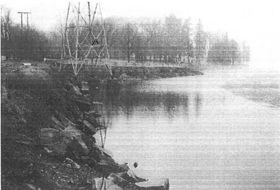
Photo B8: View from the right abutment of the dike.
