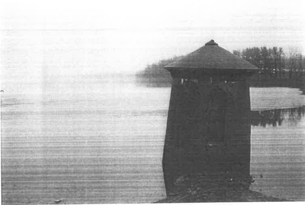
Photo B5: Abandoned Gate house
