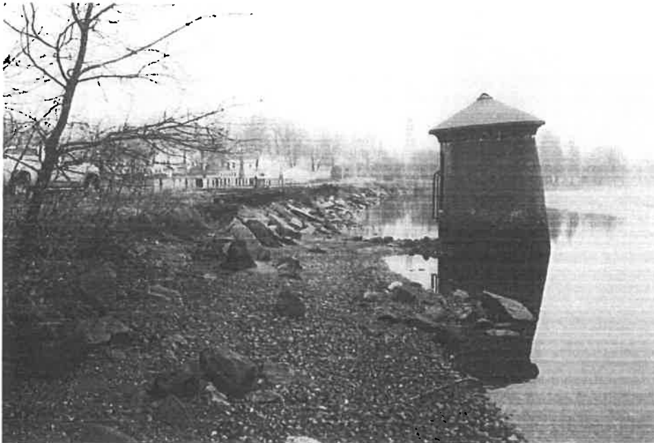
Photo B4: View of the dike upstream slope protection.
