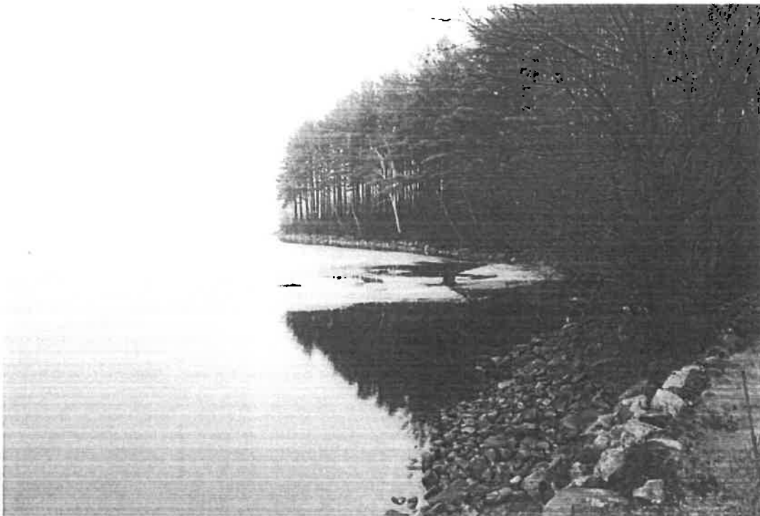
Photo B12: View of the left abutment
