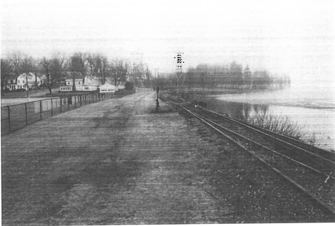
Photo B1: View of the dike crest looking towards the right abutment.
