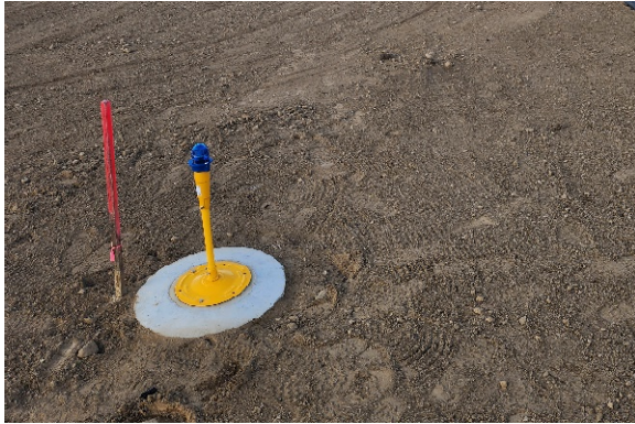
Figure 2-6: Newly Installed Taxiway Light
