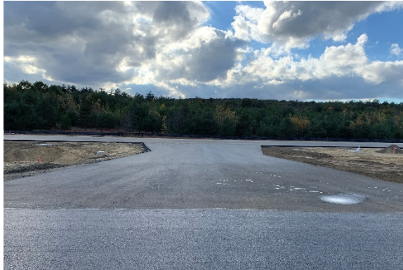
Figure 2-4: Newly Constructed Stub Taxiway
