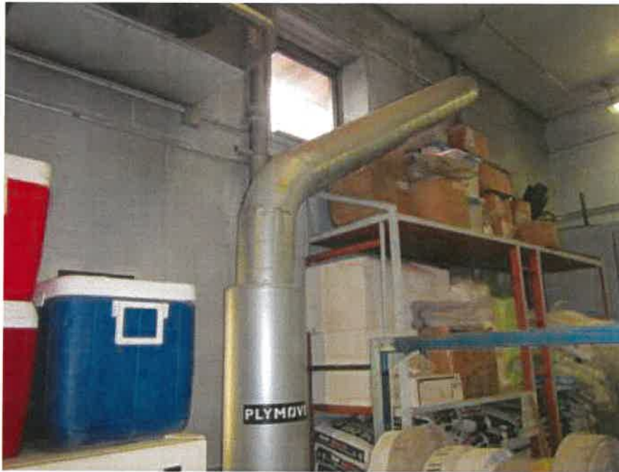
Plymovent™ vehicle exhaust system
