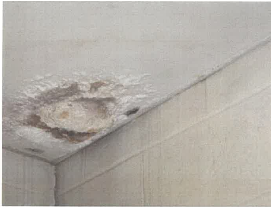
Water-damaged ceiling in upstairs locker area
