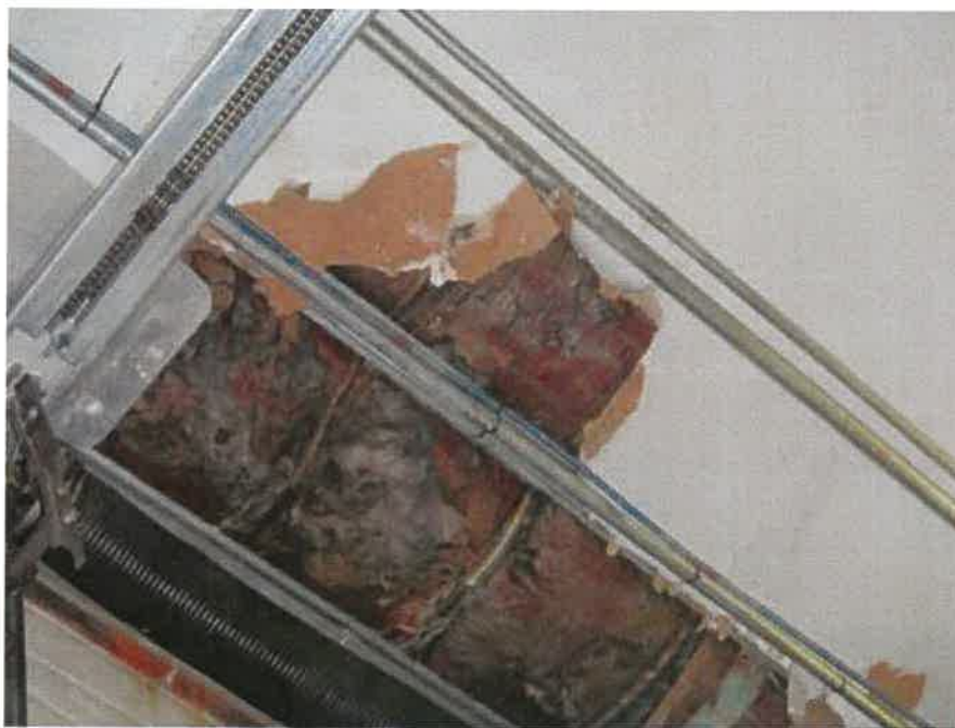
Water-damaged ceiling in the apparatus bay
