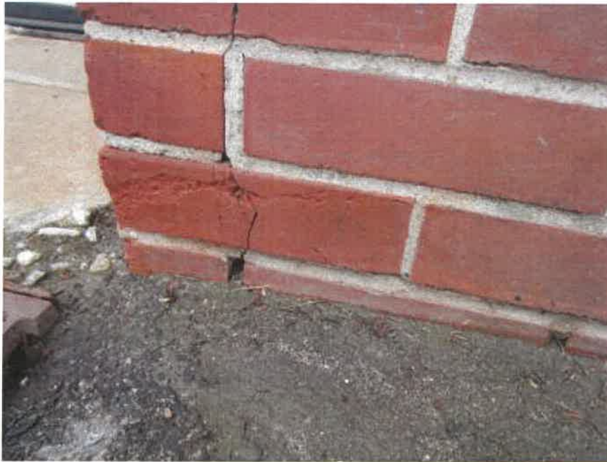
Building exterior; note partially obstructed weep holes and cracks in brick/mortar
