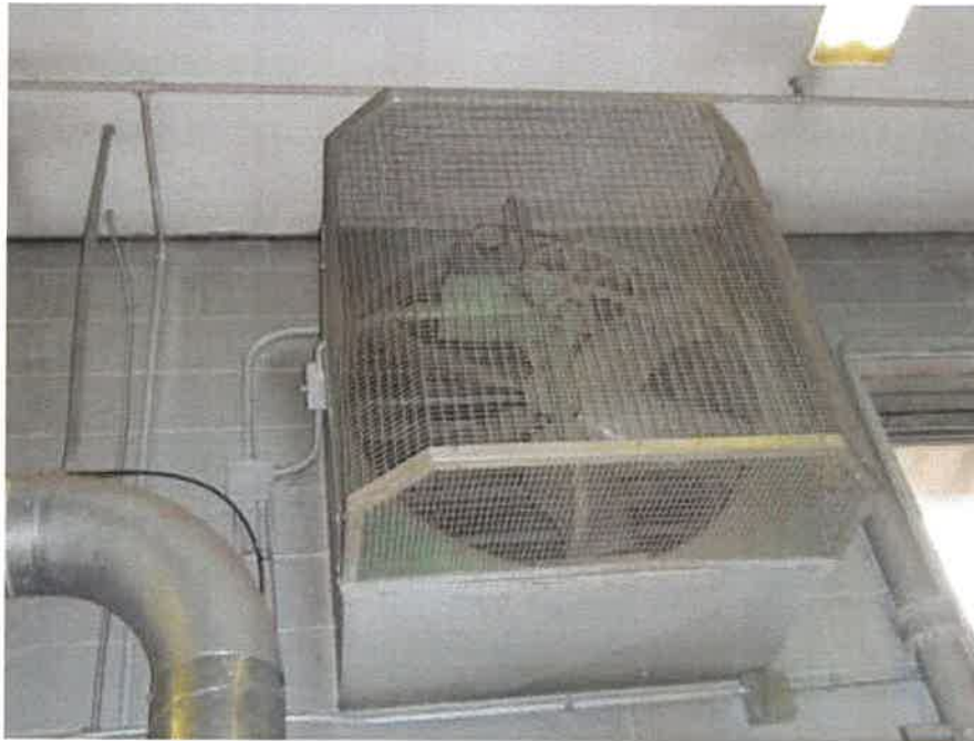
General exhaust fan in the GFD apparatus bay
