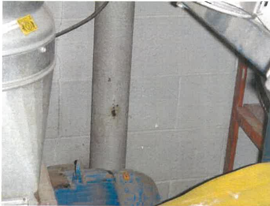
Single drain serving each side of roof/gutter system
