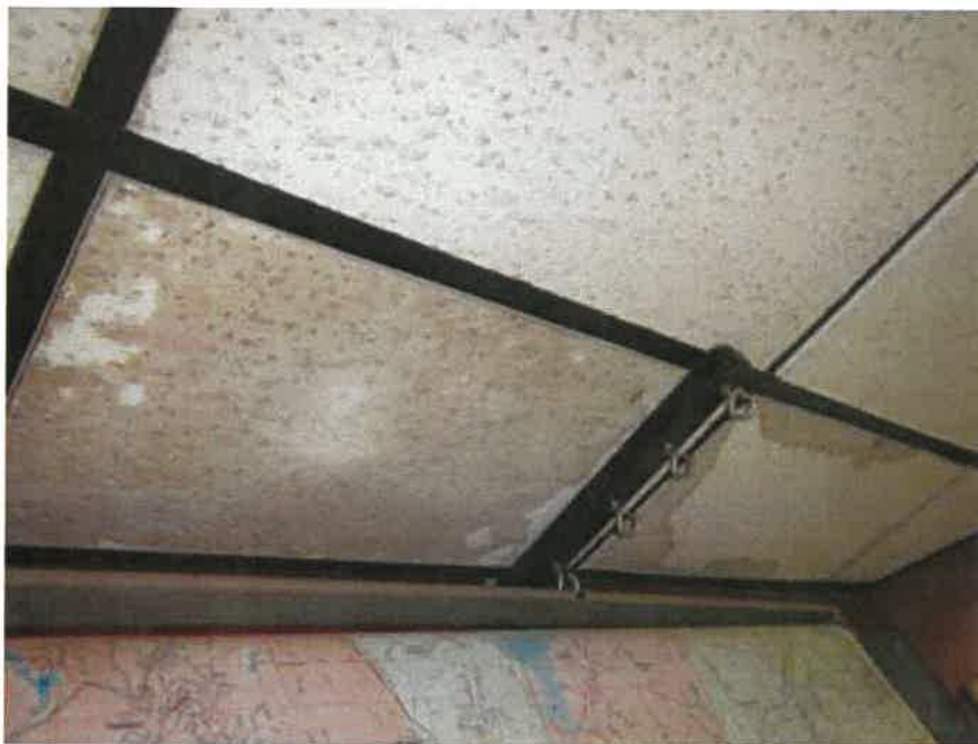
Water-damaged ceiling in the dispatch area
