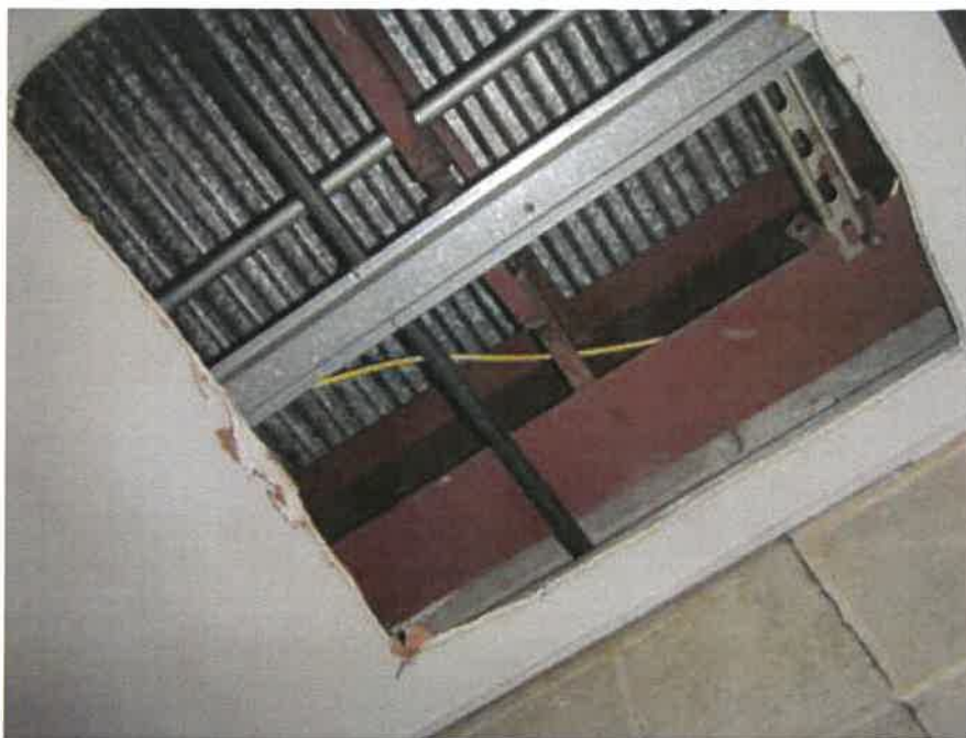
Large hole in mechanical room
