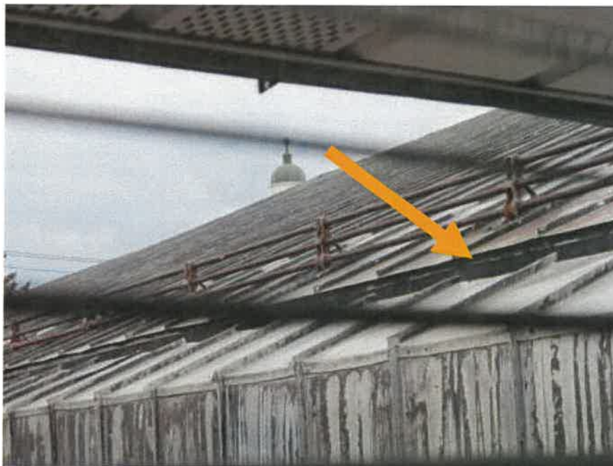
Roof showing “embedded” gutter system
