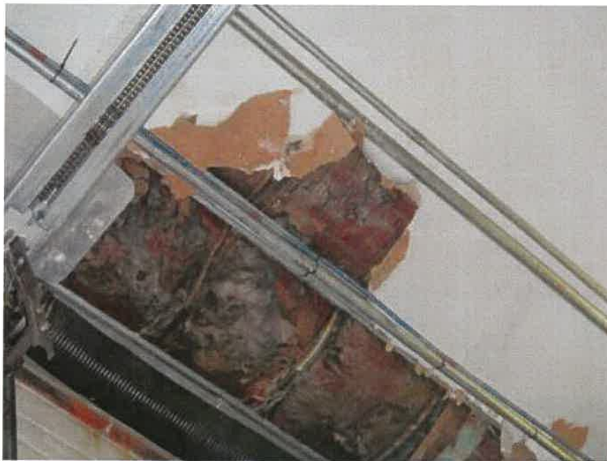
Water-damaged ceiling in the apparatus bay
