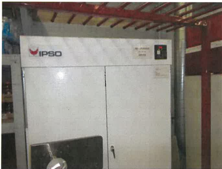
Turnout gear dryer not vented to the exterior
