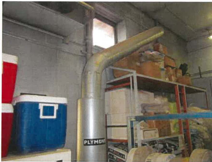
Plymovent™ vehicle exhaust system
