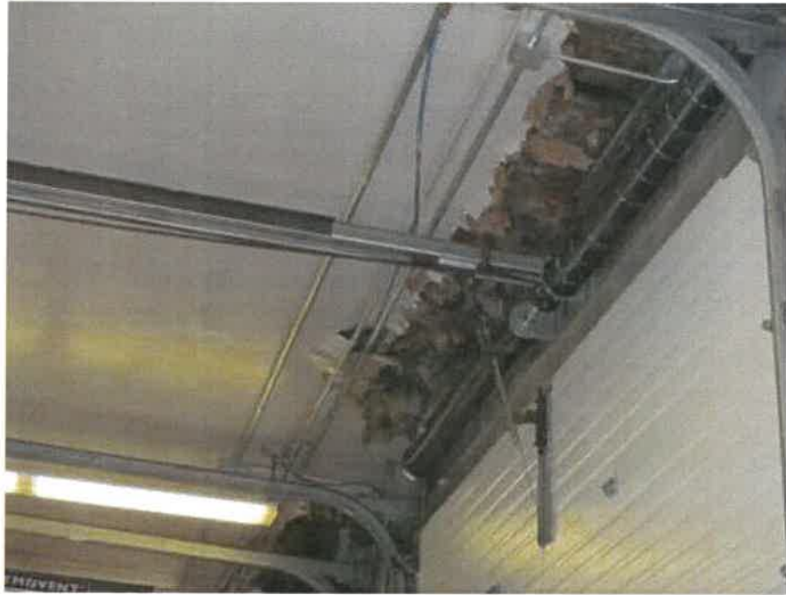
Water-damaged ceiling in apparatus bay
