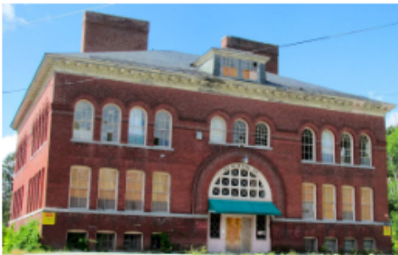
School Street School
