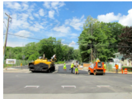
Paving Pearl Street entrance
