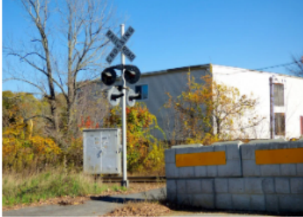
South Main Street Bridge near Railroad
