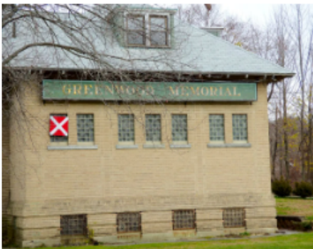
Greenwood to be Torn Down
