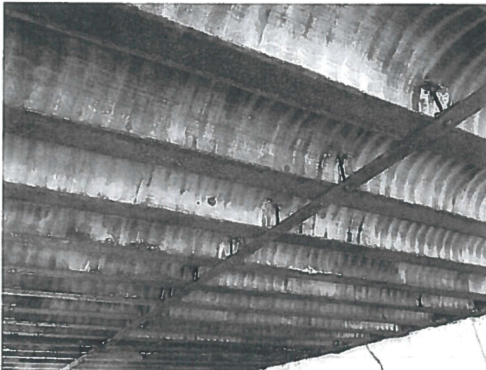
Photo 6: Typical condition of the beams away from the North abutment.
