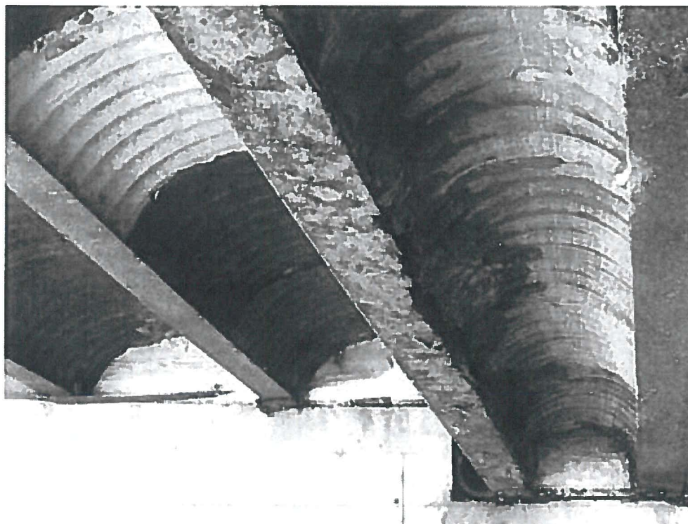
Photo 4: West edge of the bottom flange of beam #25.
