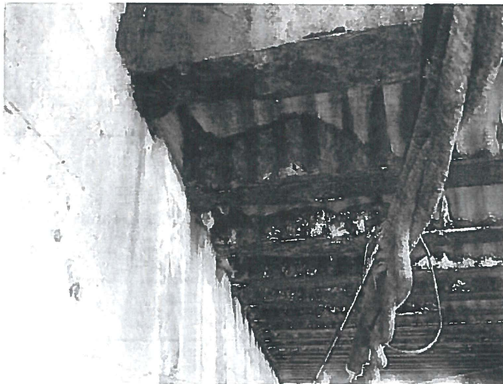
Photo 5: Typical North ends of the beams.
