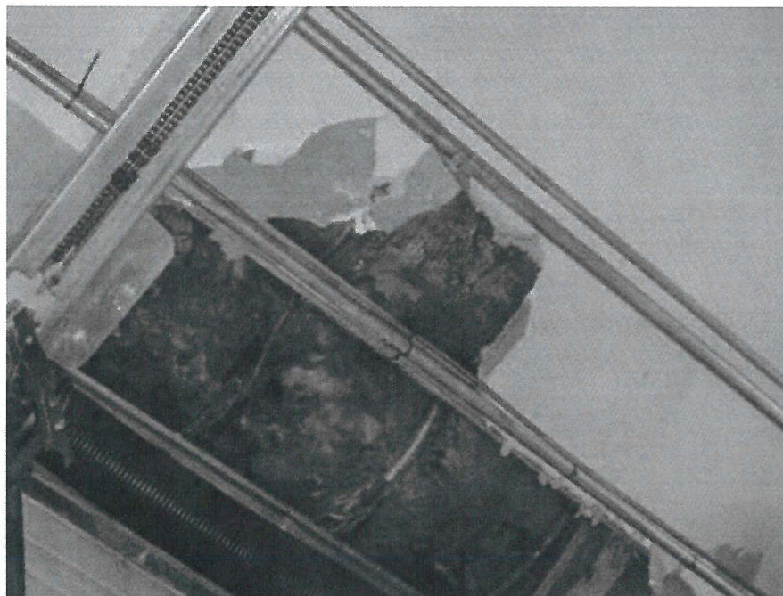
Water-damaged ceiling in the apparatus bay
