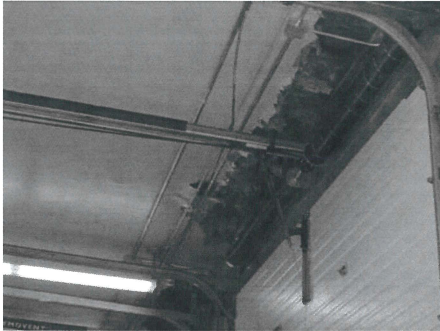
Water-damaged ceiling in apparatus bay
