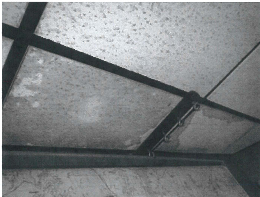
Water-damaged ceiling in the dispatch area
