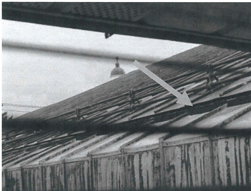
Roof showing “embedded” gutter system
