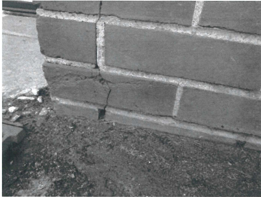
Building exterior; note partially obstructed weep holes and cracks in brick/mortar
