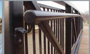
Vertical Picket/Pipe Handrail
